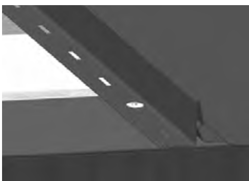
Figure 15. Correct screw tightness
