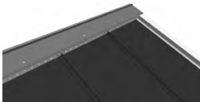
Figure 32. Installing the ridge capping
