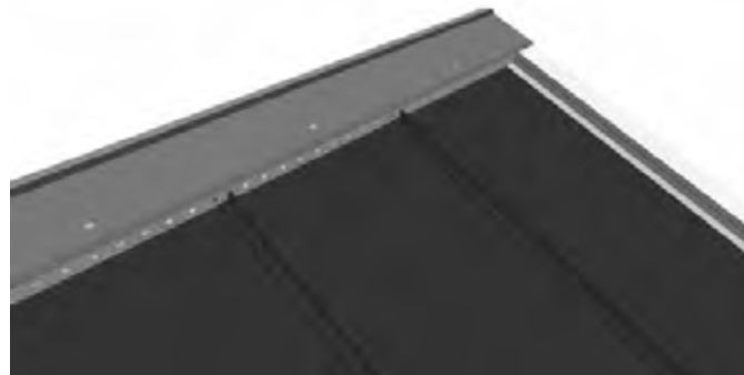
Figure 32. Installing the ridge capping
