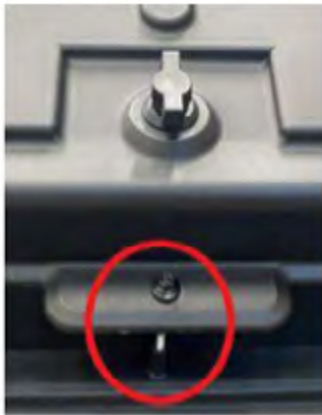
Figure 49. Hatch locked and secured with a screw
