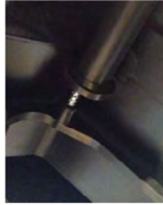
Figure 48. Properly placed screw
