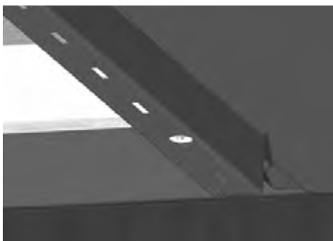
Figure 15. Correct screw tightness
