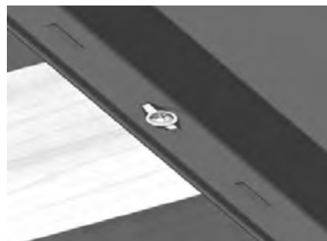
Figure 16. A screw that is too tight
