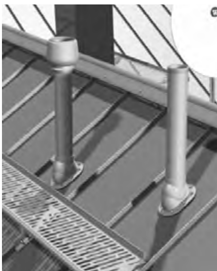
Figure 39. The placement of penetration elements on the pane of the roof
