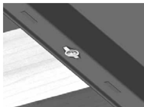
Figure 16. A screw that is too tight
