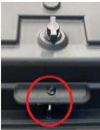
Figure 49. Hatch locked and secured with a screw
